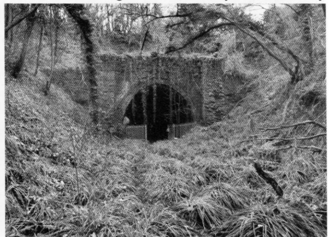
The south portal of Etchinghill Tunnel in March 2012. Photo Nick Catford
